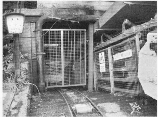
Drift exit from Caphouse, showing conveyor belt. Photo by Linda Bartlett
